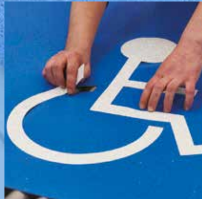
Sections can be moved easily into place.
