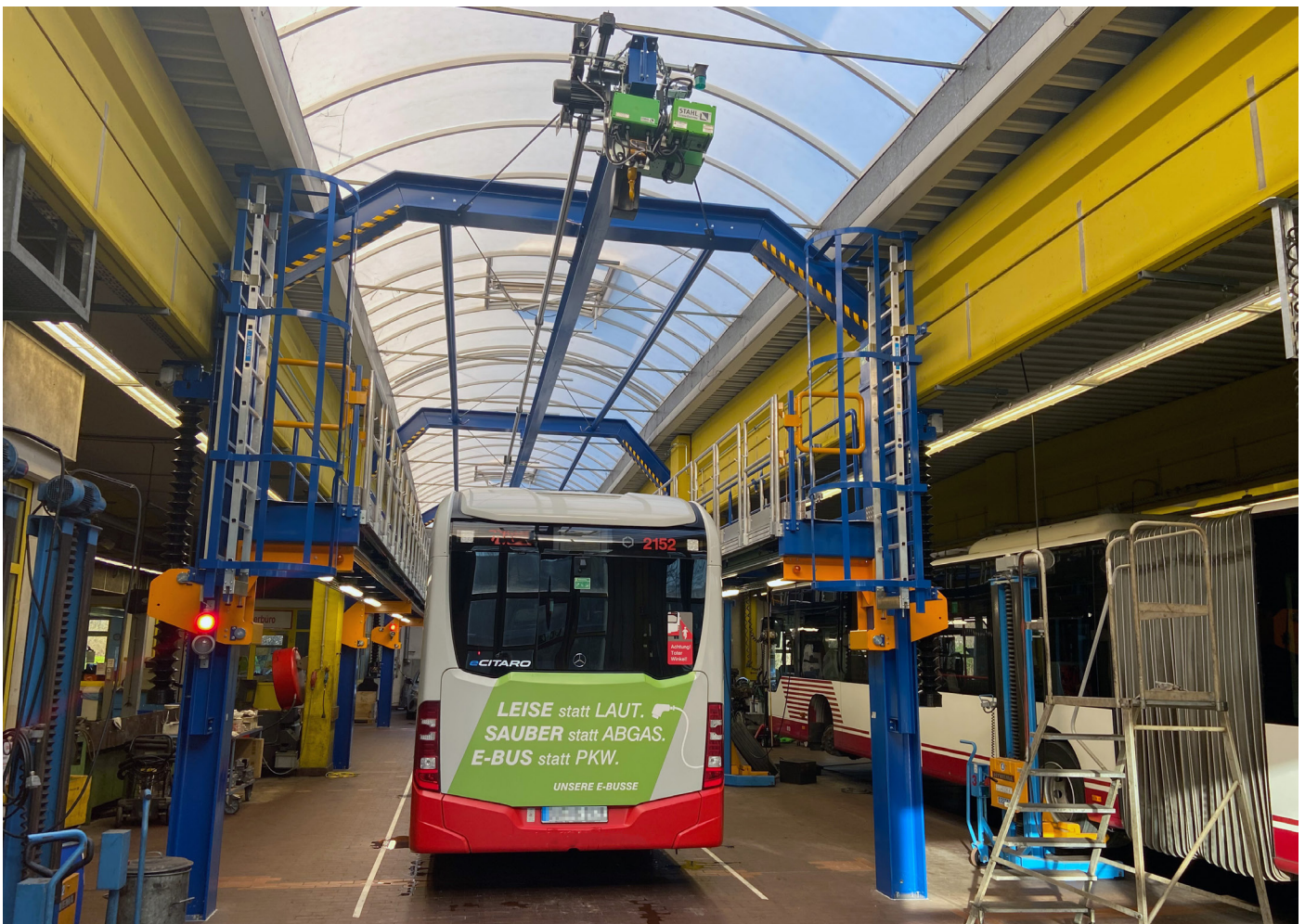
The roof-working platforms from Pfaff-silberblau on the side & the crane from STAHL CraneSystems above are a very common combination among customers
