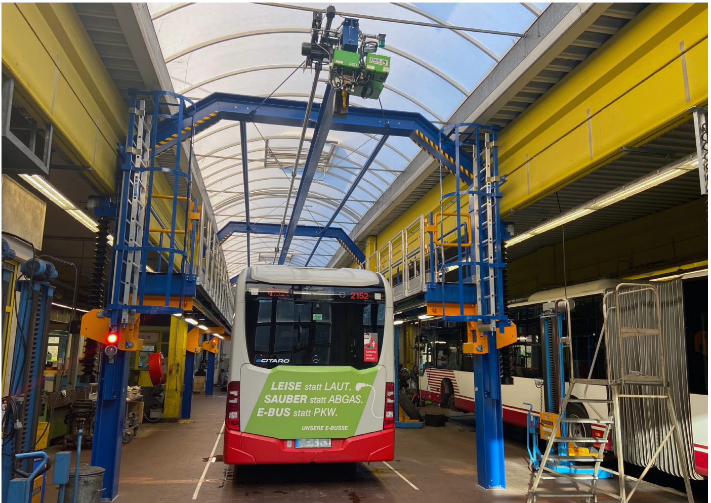
The roof-working platforms from Pfaff-silberblau on the side & the crane from STAHL CraneSystems above are a very common combination among customers
